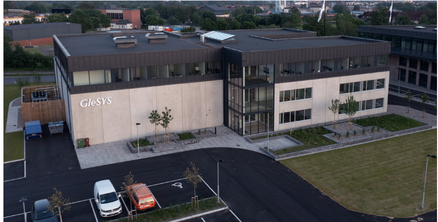
Figure 10 – GleSYS Facilities in Vastberga, Stockholm, Sweden
